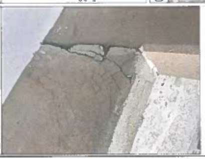
11.4 DETAILING OF RETAINING WALL PHOTO
